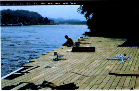
overstroombare houten kaai floodable wooden quayside
