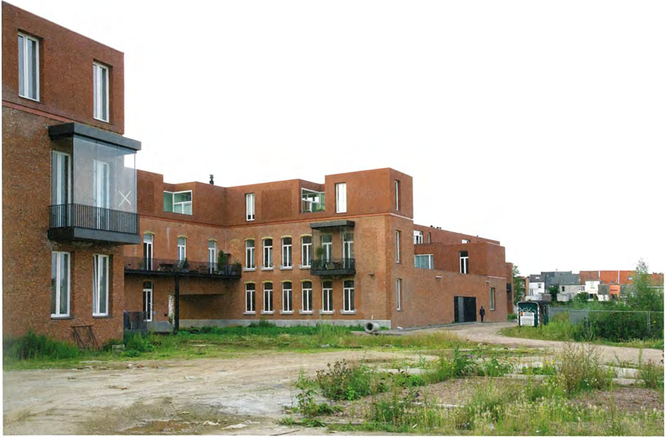
In the central section all the listed historic buildings are given a facelift. Additional floors are provided on the roof.
